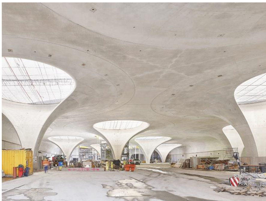
Ilustración 16 - Estructura Main Station Stuttgart. Fuente: https://www.wernersobek.com/wp-content/uploads/resized/2020/05/S21-in-Stuttgart-Kelchstutzen-1-1920x0-c-default.jpg
