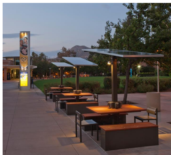
Ilustración 58. Off-grid Solar-Powered Charging Stations. (Innes, J., 2017)
