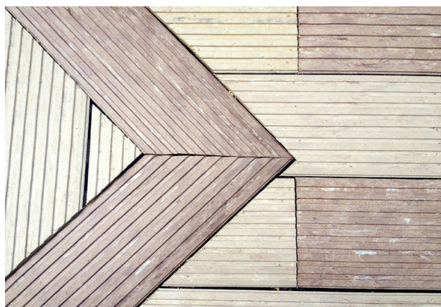
Deck en eco-deck hard.
