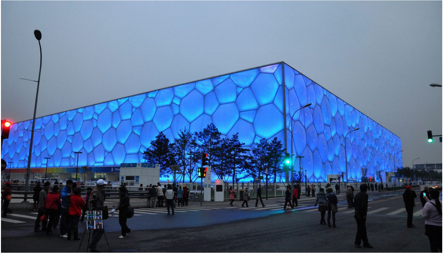
Figura 24: Beijing's Water Cube
