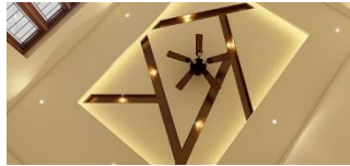
photo of ceiling:
